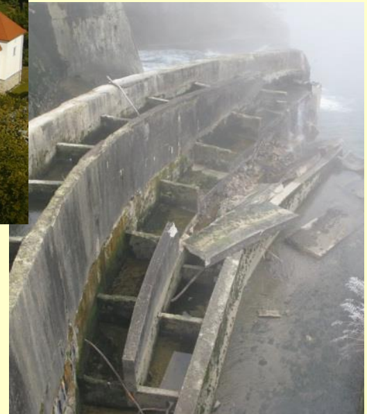
Collapse of the fish pass No.1 in November 2013 due to high water discharge
