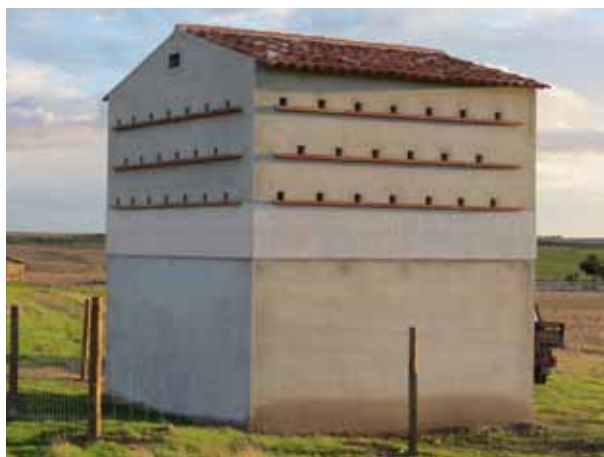
One of the two breeding towers the project constructed to boost the lesser kestrel population
