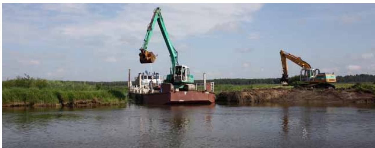
Working to reconnect an oxbow lake and the main course of the Emajõgi river
